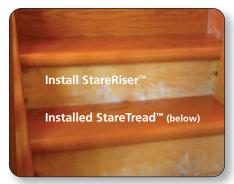
Working down, install the StareTread first, then the StareRiser above
